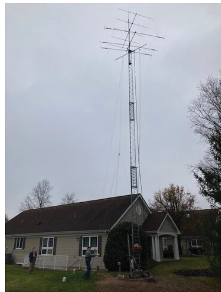
Tom W3EX and Dan WA3NFV working toward successfully elevating the 160/80/40 Meter Dipole on the K3PBC Tower.
