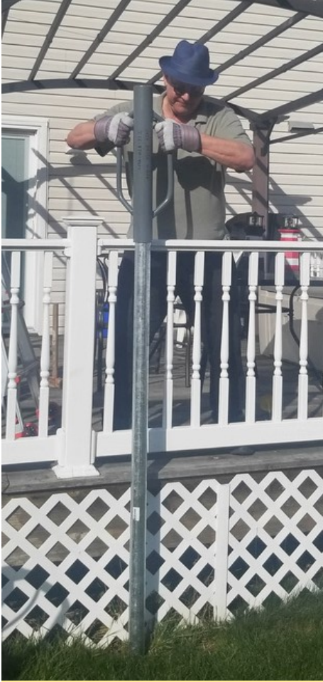
Installing the support pipe.
