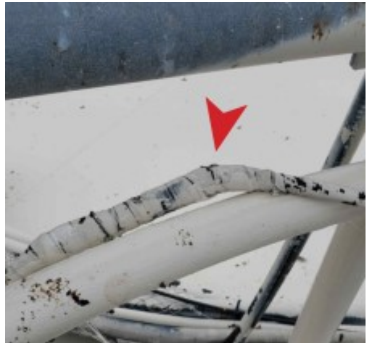
Damaged splice from Hardline to Superflex jumper. Note the red arrow.
