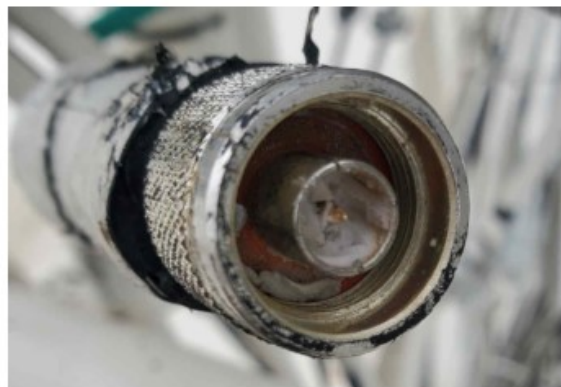
Dielectric in splice - Removed!
