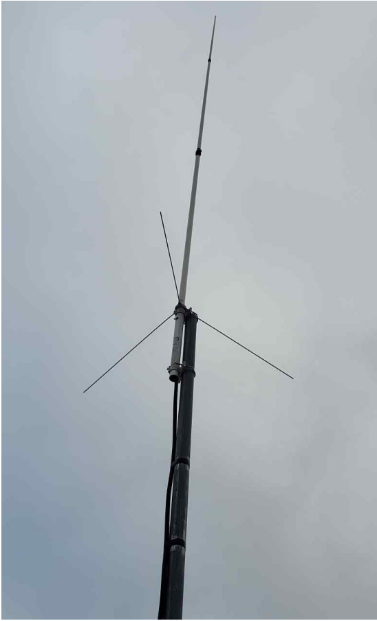
2M Repeater Antenna atop water tank.
